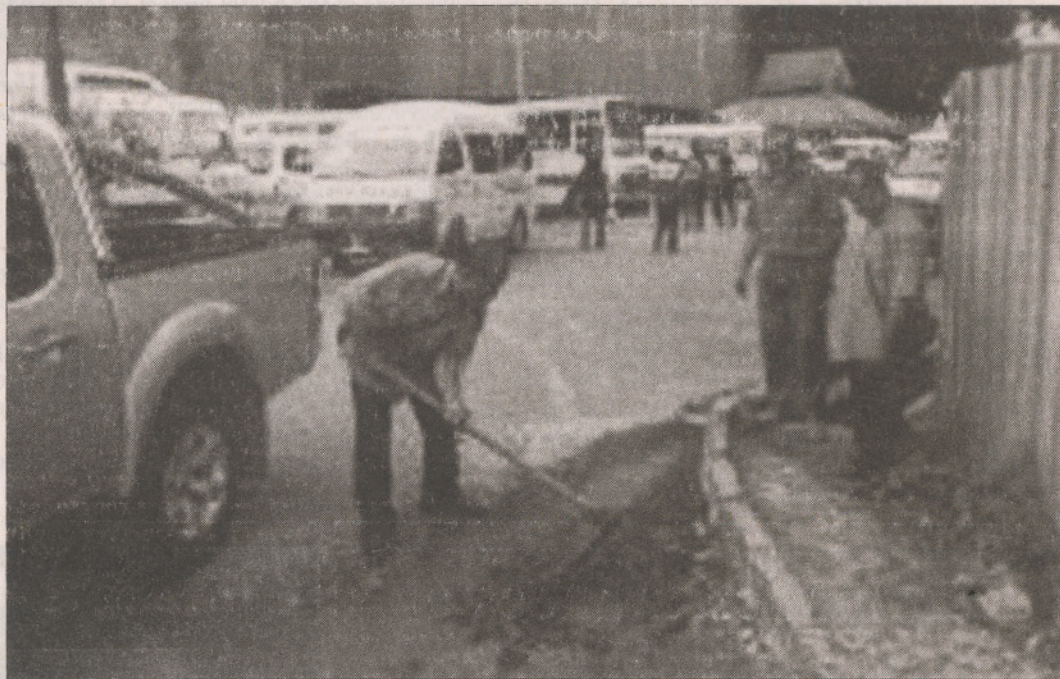
Bus drivers repairing a pothole at the bus terminal in Labuan.
